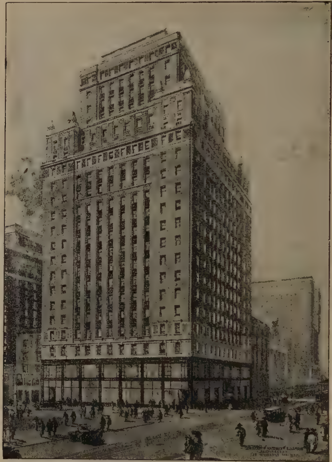
465 Carrère and Hastings, and R. H. Shreve, architects
